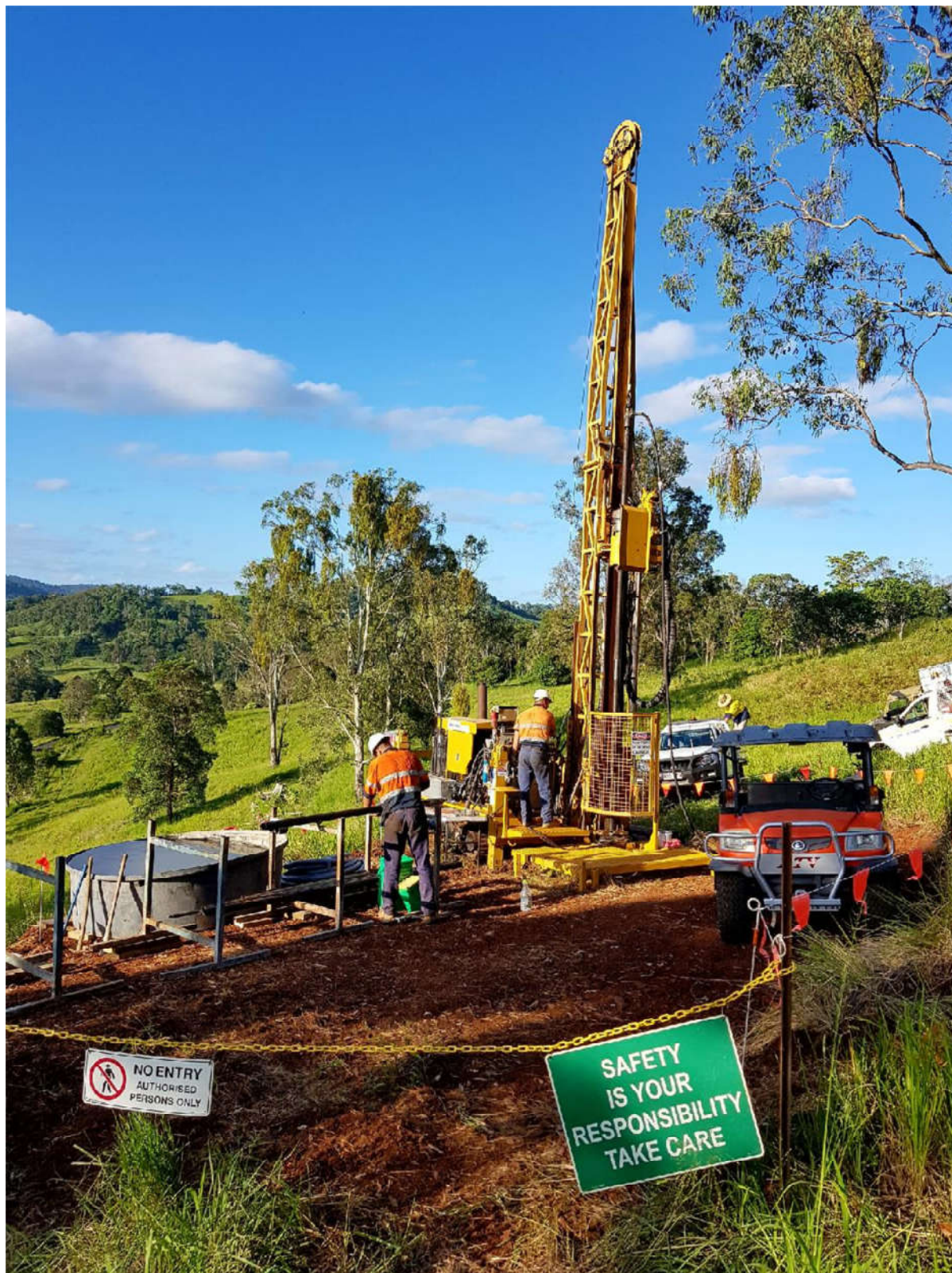
Figure 3. Diamond drill rig on site at Eel Creek
